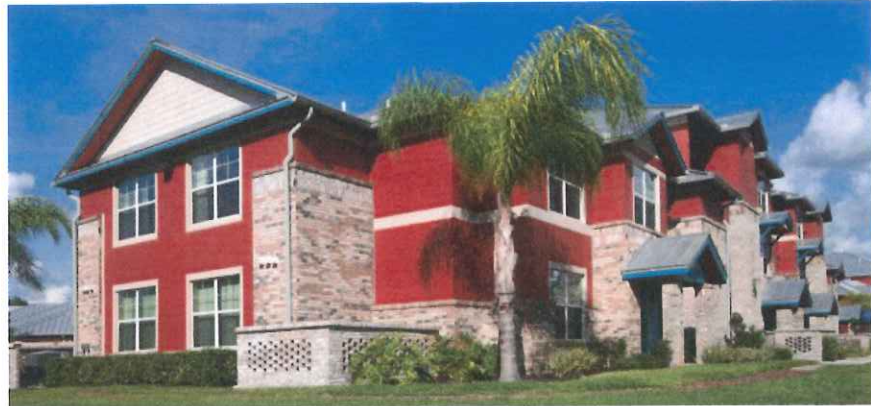
Pictured are (from top left) Poehler Lofts in Lawrence, Kan.; Oak Street Lofts in Portland, Maine; Cascade Ridge in Great Falls, Mont.; and Cypress Cove in Winter Haven, Fla.
